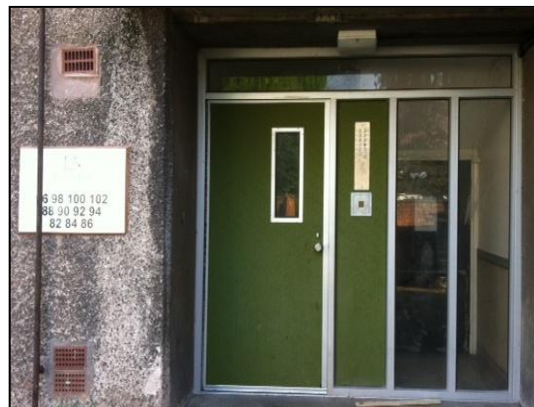
Hesketh Road, Stafford. Installed 1990
